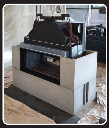
The kit is made from refractory concrete highly efficient in absorbing heat and holding on to the heat for a long time, in essence similar to floor heating within a heater structure.
